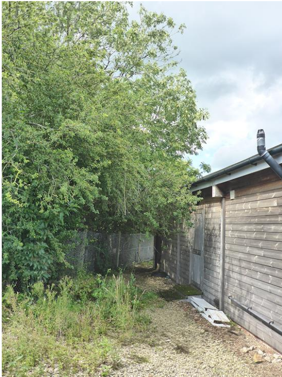
21. Mixed group: Crown lift to clear pavilion.
